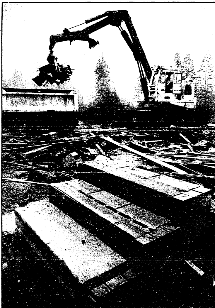
Lige Calkins loads debris from home into dump truck.
